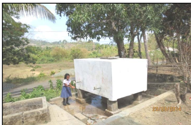
Drinking water facility in the sample school
